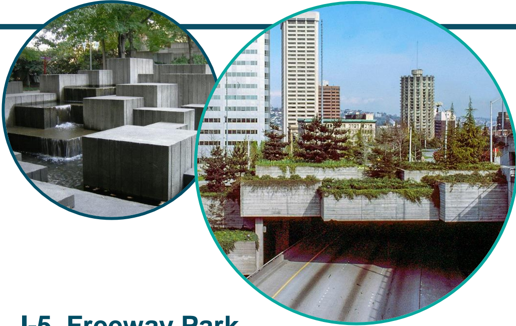
I-5, Freeway Park Seattle, Washington
