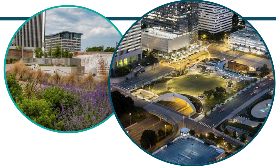
I-195, Kanawha Plaza Richmond, Virginia
