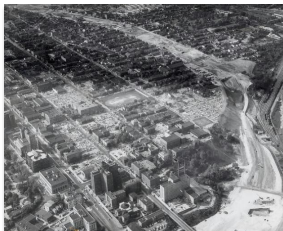
Aerial view of construction of the Richmond-Petersburg Turnpike in Jackson Ward
